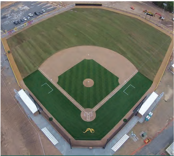
A synthetic turf infield can help to extend the play time on a field due to quick recovery times after a rain event.
